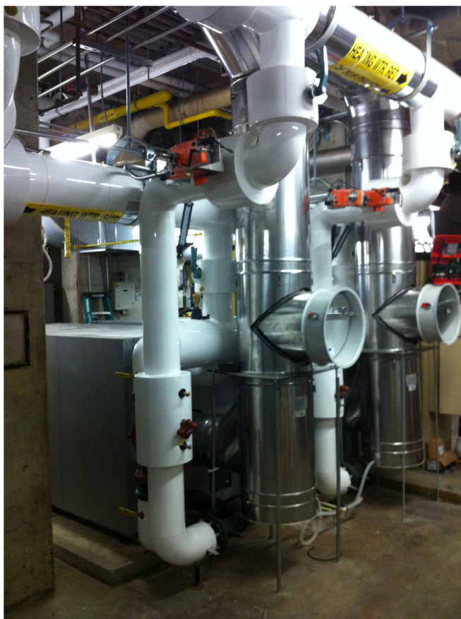
New Domestic Heating Boilers in Saugeen-Maitland Hall
