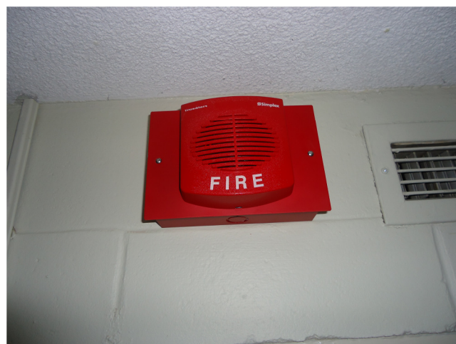
New in-room fire alarm speakers at Saugeen
