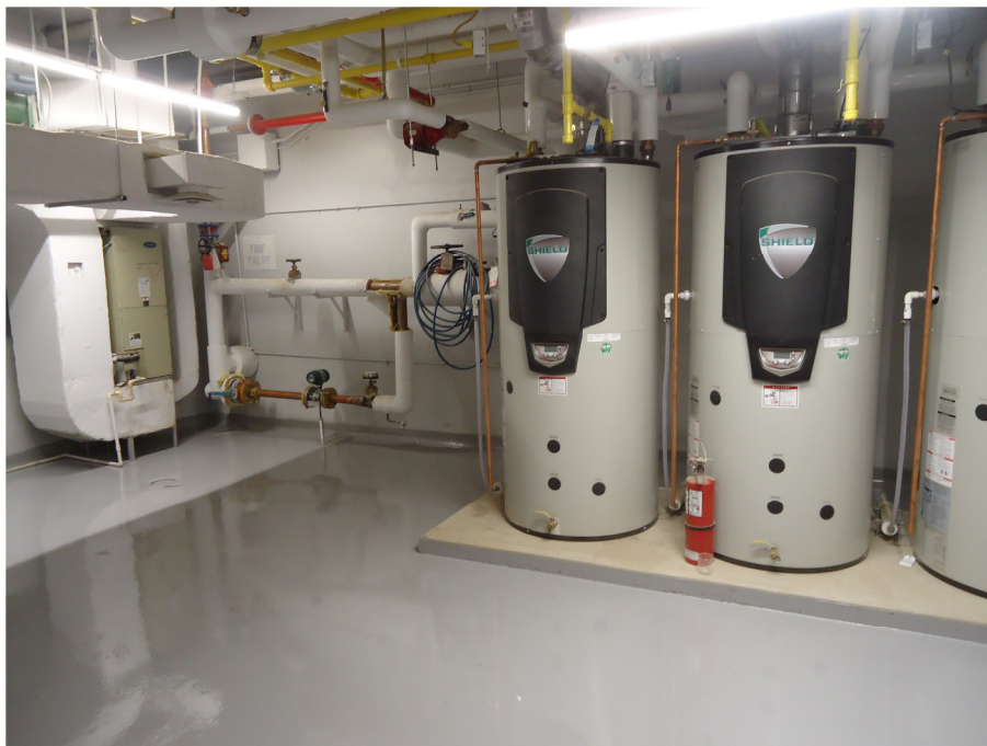
New Domestic Heating Boilers – Sydenham
