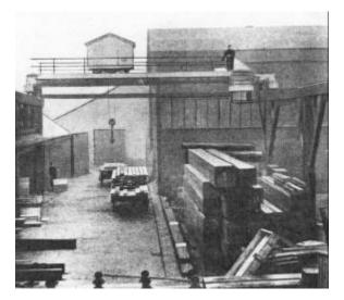
Overhead Travelling Crane at Miles Platting Mill, 1907.<sup>66</sup>
