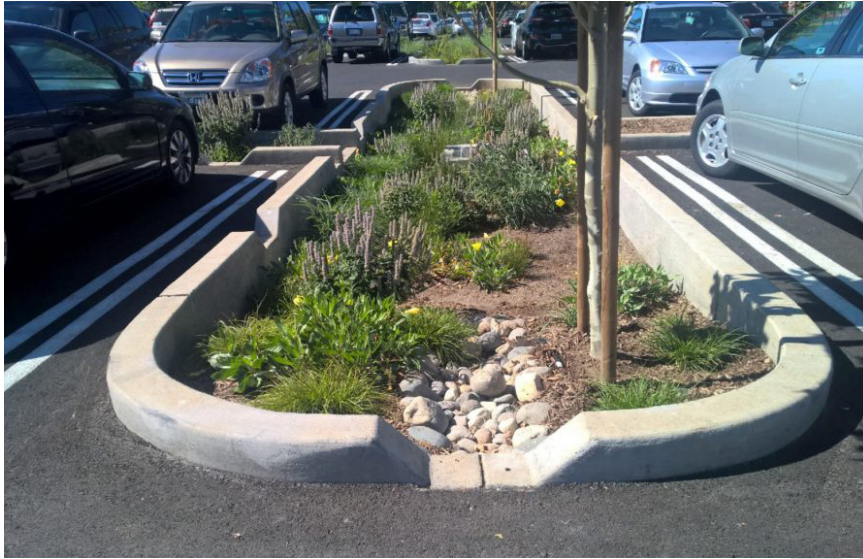
Examples of curb cuts and drainage swales channel which would allow rainwater to infiltrate into planting areas during rain events.
