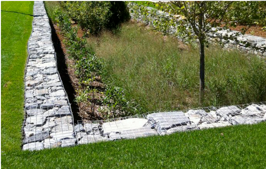
Example of an infiltration bed, allowing rainwater to collect and infiltrate.
