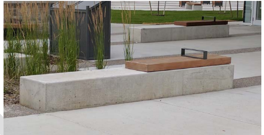
Elements can be incorporated into seatwall design that enhance the wall while deterring use by skateboarders.
