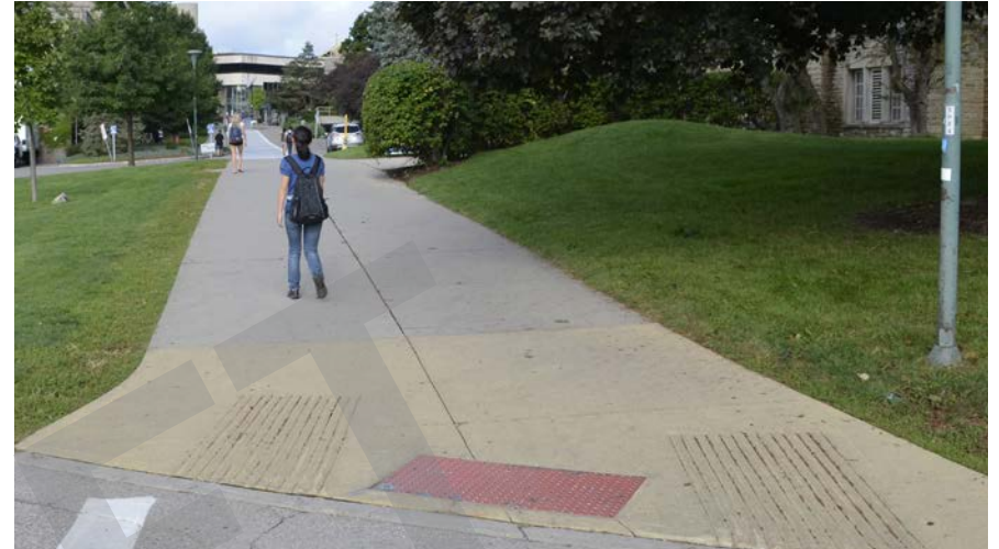
The bright red plates and yellow concrete ramps located at the edge of road crossings provides aid for the visually impaired.
