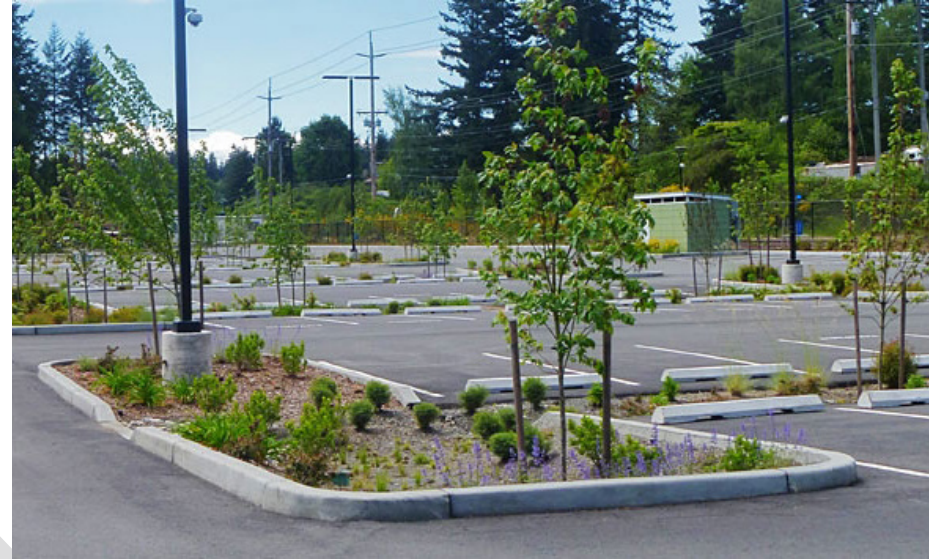
Examples of curb cuts and drainage swales channel which would allow rainwater to infiltrate into planting areas during rain events.
