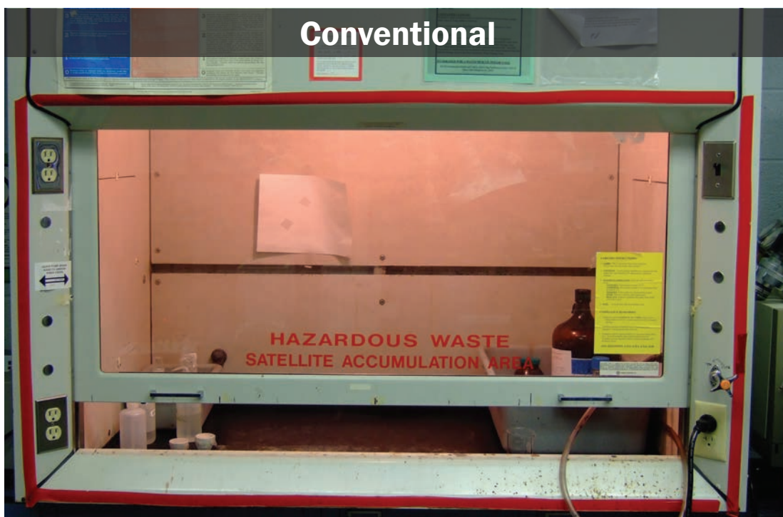
Figure 10. Conventional (constant-flow) laboratory chemical hood.
