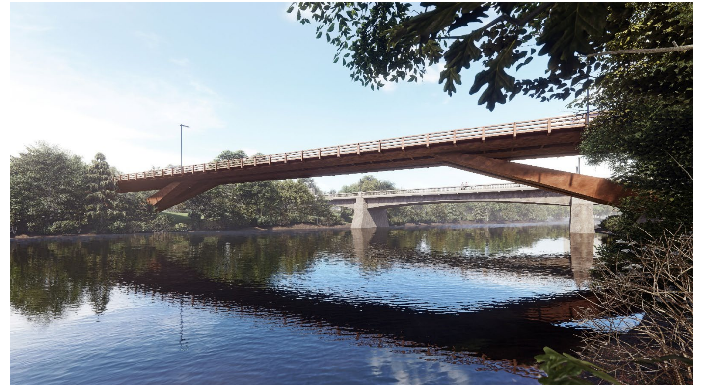
Figure 17: Steel V-Pier Bridge Alternative
