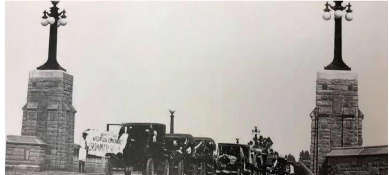
Photo 1: Original Bridge Opening
