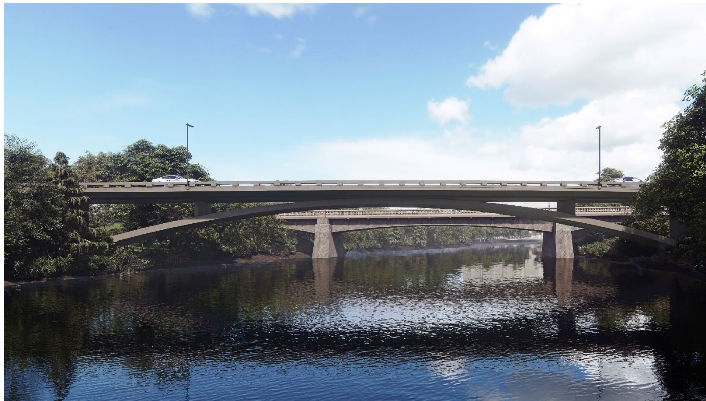
Figure 16: Concrete Arch Bridge Alternative
