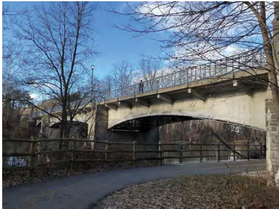
Image 8: View of south side of bridge, looking north; note steel cross bracing visible from open barrel arch (WSP, 2018).
