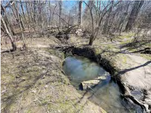
Culver Outlet No. 6 (above) is located approximately 20 m north of the bridge. The outlet shows signs of severe erosion, appears to contain water year-round, and bisects the trail without a formal crossing structure (below).
