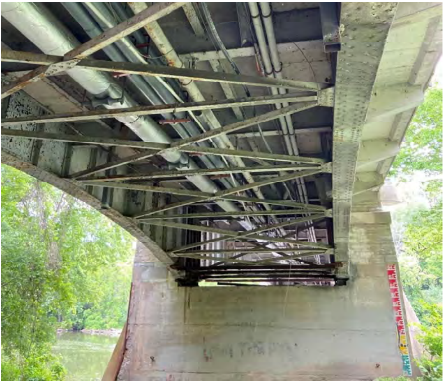
Figure 8: Major Utilities on the Underside of the Bridge
