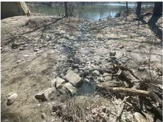
Culvert Outlet No. 3 (above) does not have a particularly well-defined channel (below). Riprap and cobble have been placed as an interim repair method. Standing water was grey and likely untreated upstream.
