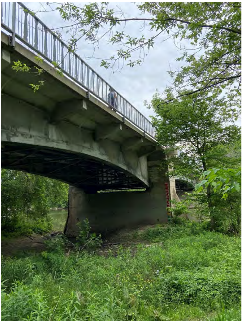
Figure 11: View of University Drive Bridge from Below Illustrating Decorative Concrete on the Outside of the Steel Girders
