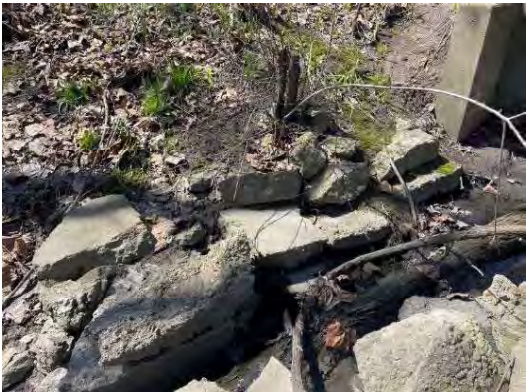
Riprap material appears to have been placed along the banks of the outlet channel in an attempt to reduce erosion (above). However, erosion issues persist (below).
