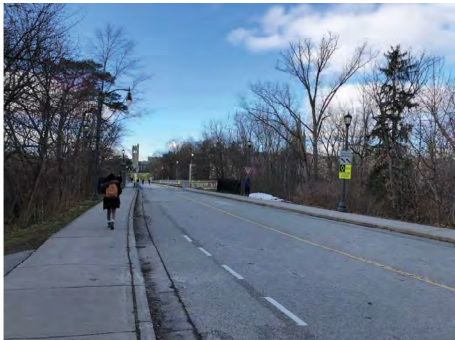
Image 2: East approach to University Bridge, looking west (WSP, 2018).
