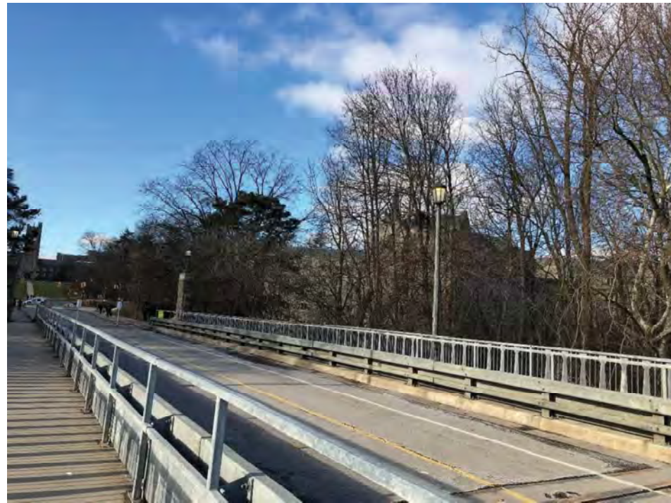
Image 16: View looking northwest on bridge, note railing between sidewalk and road surface's design (WSP, 2018).
