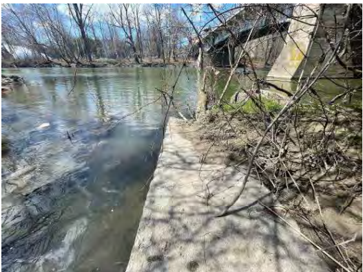
The culvert appears to have at one time had a concrete spillway (above) which is now partially damaged and showing signs of erosion (below).
