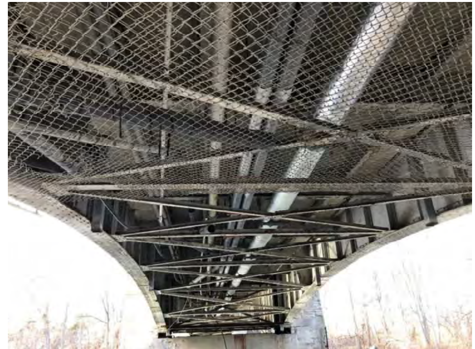
Image 11: View of the eastern most span of the bridge, looking west (WSP, 2018).
