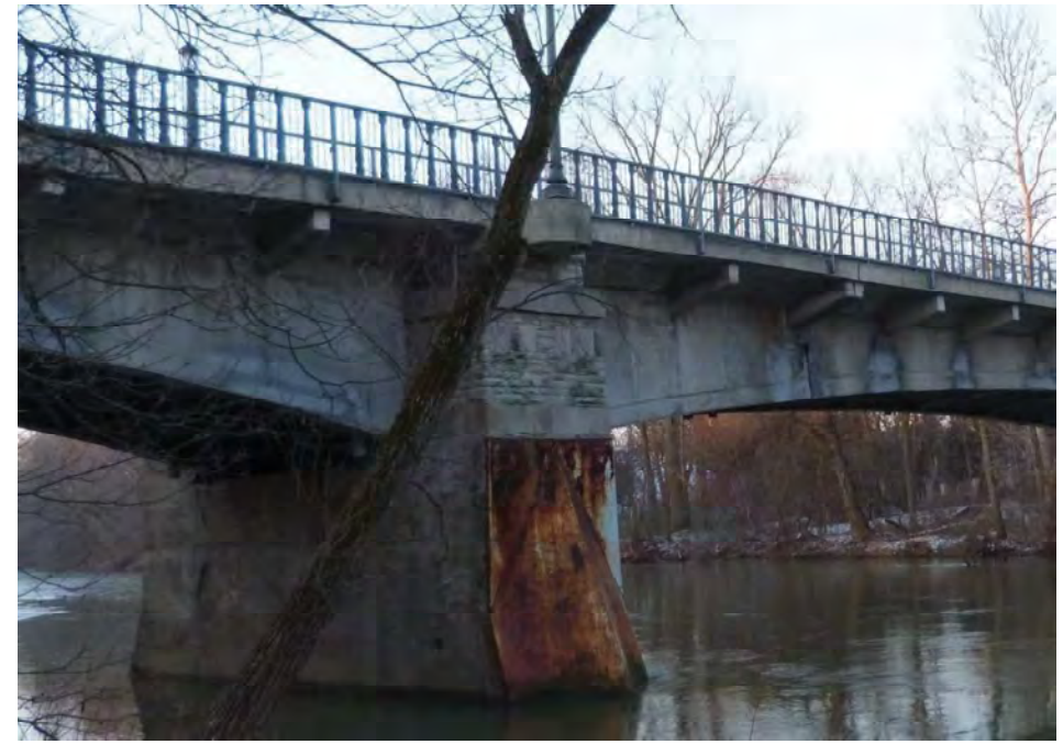
Image 10: Detail of concrete and stone pier, looking south, note shield shaped stone (WSP, 2018).
