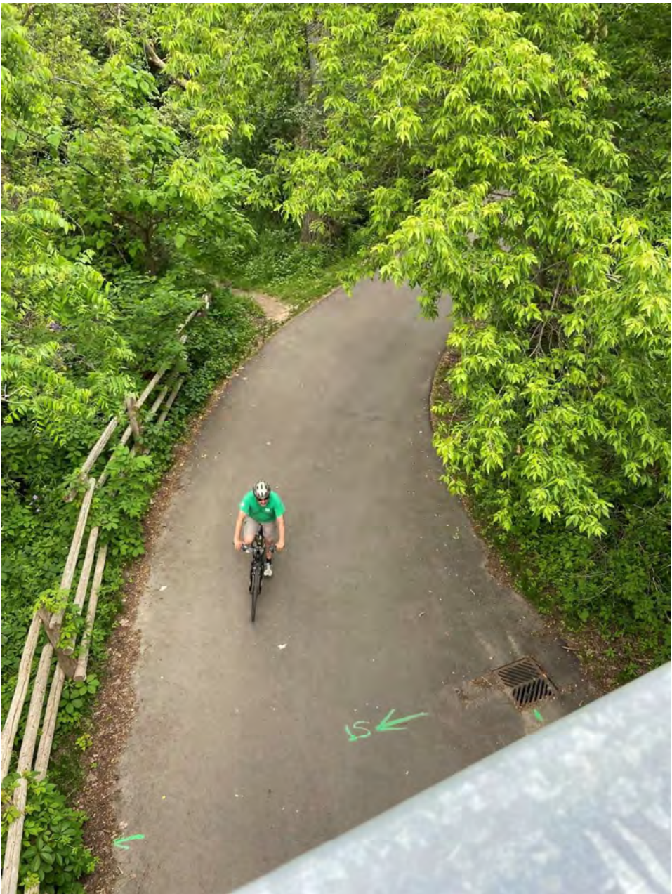
Figure 9: A paved Multi-use Path is Located under the East Side of the Bridge
