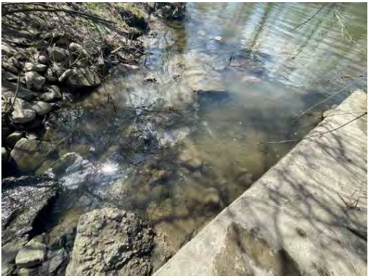
The culvert appears to have at one time had a concrete spillway (above) which is now partially damaged and showing signs of erosion (below).
