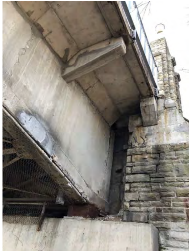
Image 13: Detail of reinforced concrete brackets supporting sidewalk on underside of west end of bridge, looking west (WSP, 2018).
