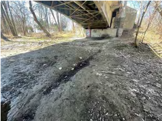
One of numerous bridge deck drains (above) outletting below onto the banks of the river (below).
