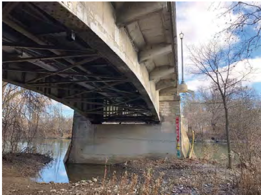
Image 9: View of the western most pier of bridge, looking east (WSP, 2018).
