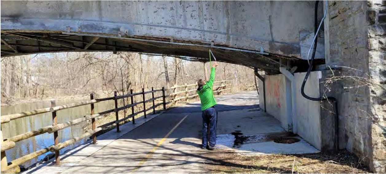
Photo 1: Measuring the Existing Clearance
