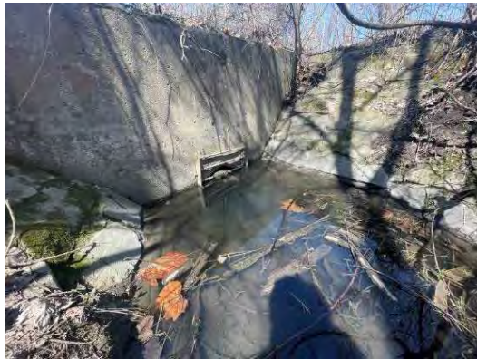
View approaching Culvert Outlet No. 3 (above) and close-up of the outlet itself, below. Note that stone walls line the outlet channel in this area (above and below).
