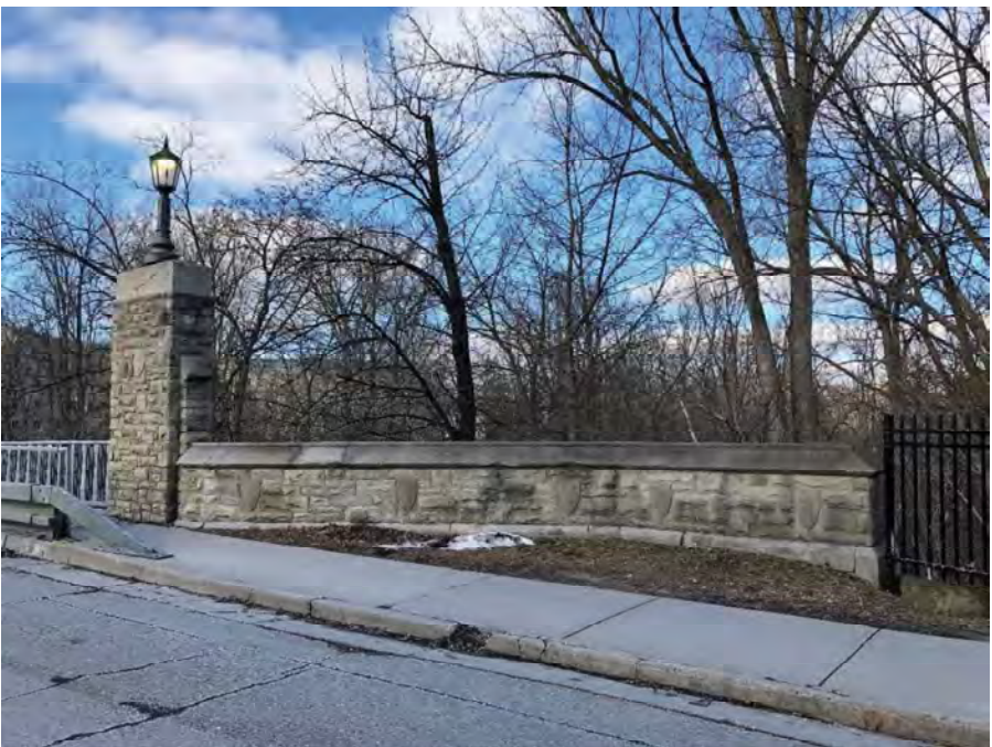
Image 4: View of north east wingwall, looking north west, note stone shields (WSP, 2018).
