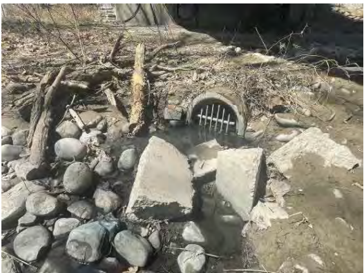
Culvert Outlet No. 3 (above) does not have a particularly well-defined channel (below). Riprap and cobble have been placed as an interim repair method. Standing water was grey and likely untreated upstream.
