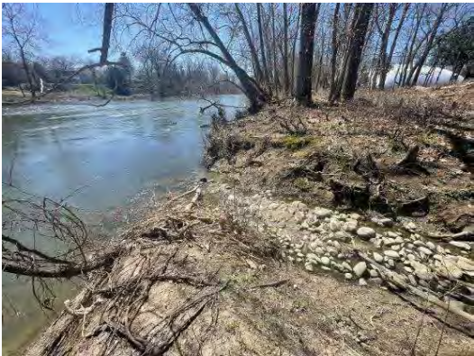
As with Culvert Outlet No. 1, this outlet channel appears to have been partially stabilized with cobble and riprap, likely in an attempt to reduce erosion (above and below).
