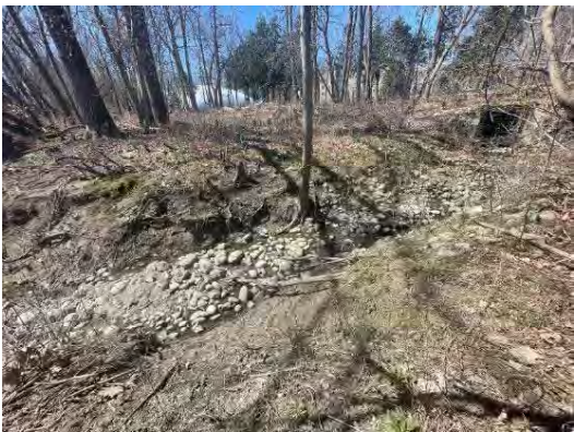
As with Culvert Outlet No. 1, this outlet channel appears to have been partially stabilized with cobble and riprap, likely in an attempt to reduce erosion (above and below).
