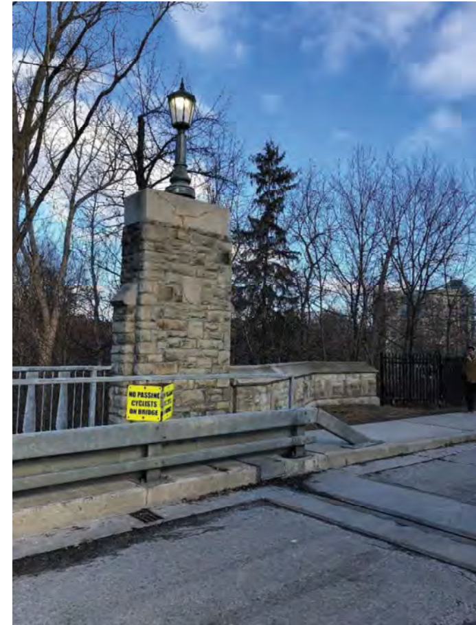
Image 7: View of north east pylon, light standard and wing wall, looking north (WSP, 2018).
