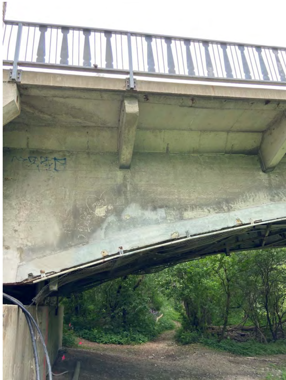
Figure 10: Sidewalk Extension on the North Side of the Bridge
