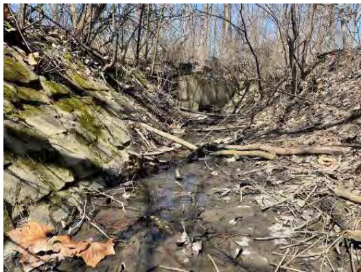
View approaching Culvert Outlet No. 3 (above) and close-up of the outlet itself, below. Note that stone walls line the outlet channel in this area (above and below).
