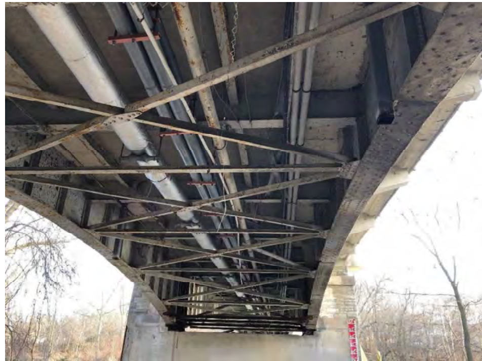
Image 11: Detail of underside of the bridge, western most span (WSP, 2018).
