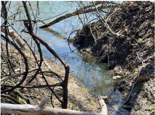
Riprap material appears to have been placed along the banks of the outlet channel in an attempt to reduce erosion (above). However, erosion issues persist (below).
