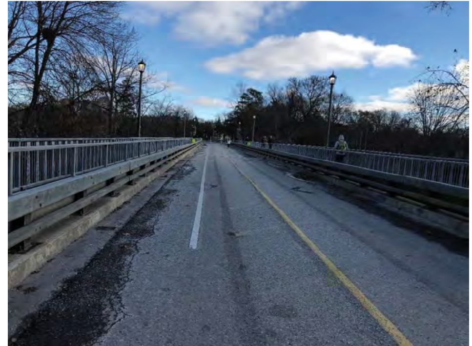
Image 14: View of road surface across bridge, looking east (WSP, 2018).
