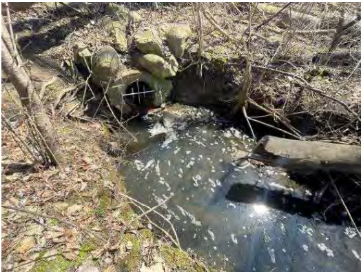
Culver Outlet No. 6 (above) is located approximately 20 m north of the bridge. The outlet shows signs of severe erosion, appears to contain water year-round, and bisects the trail without a formal crossing structure (below).
