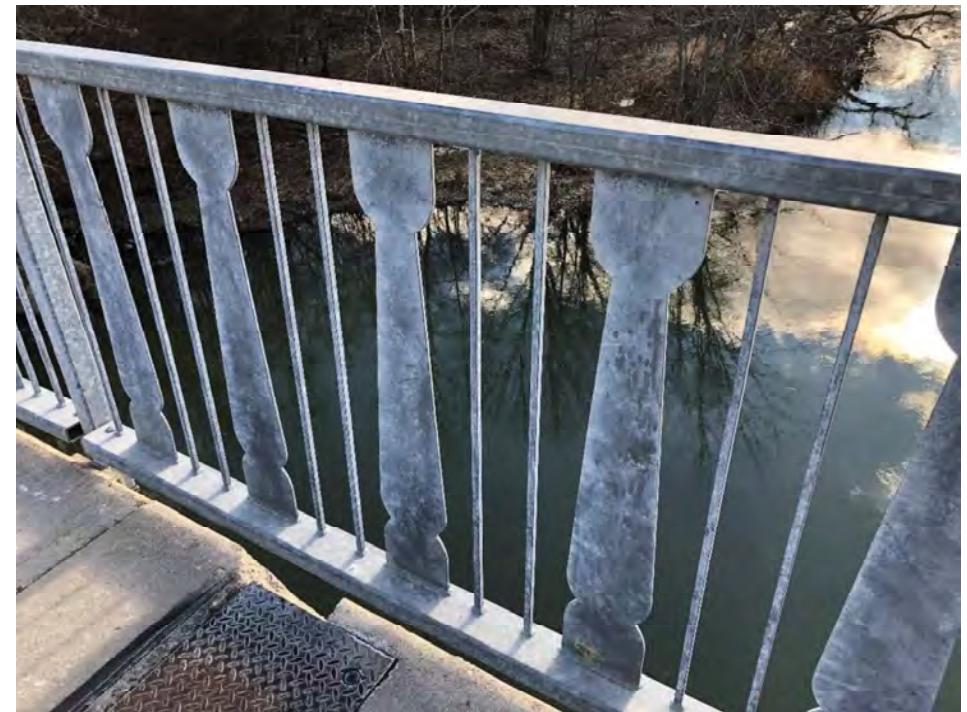
Image 15: Detail of the railing between the sidewalk and Thames River on the bridge, looking south (WSP, 2018).
