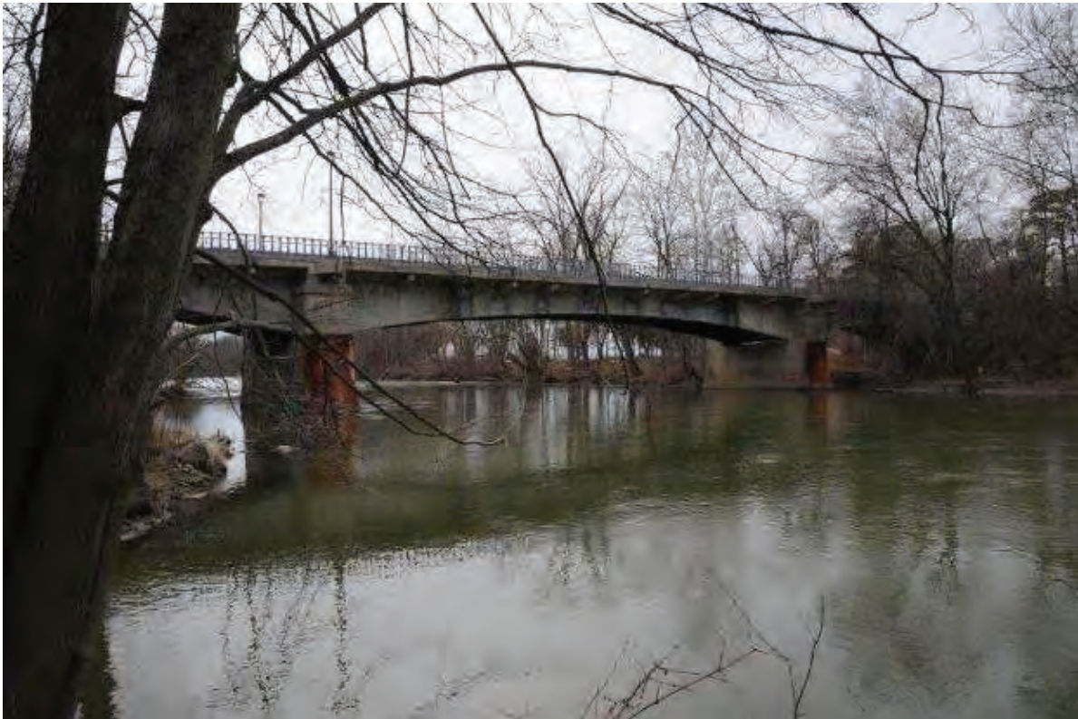
Photo 1: View of the University Drive Bridge Crossing over the North Thames River looking Southwest
