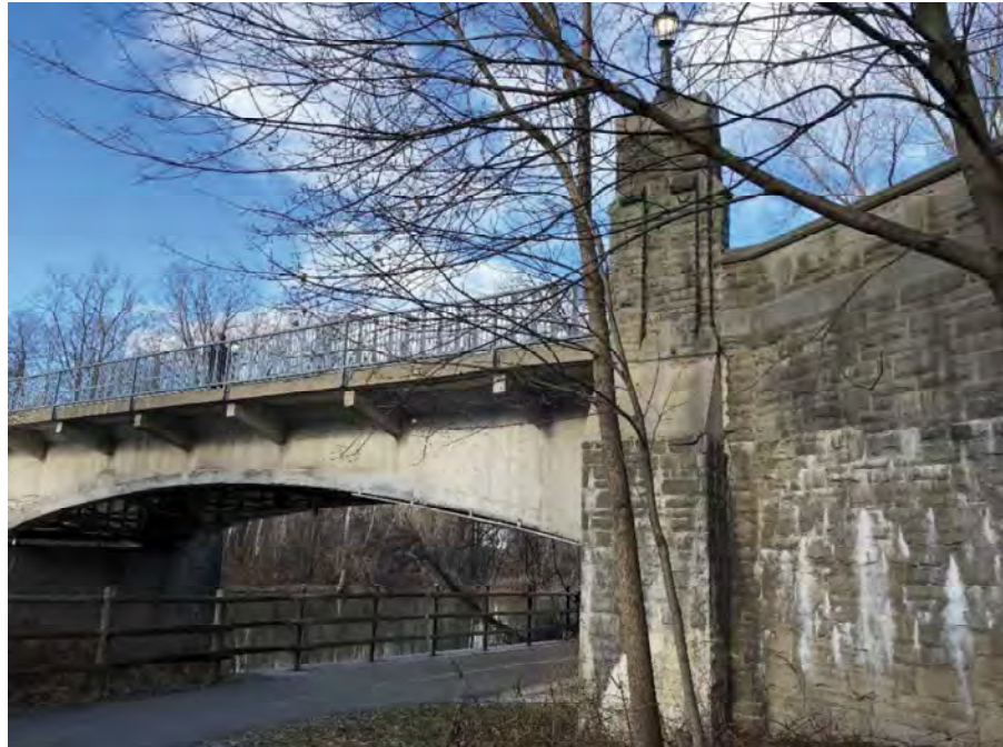
Image 6: View of toward south east abutment; note projecting buttresses on pylon (WSP, 2018).
