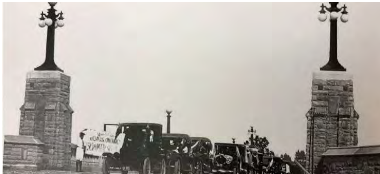
Photo 1: Original Bridge Opening
