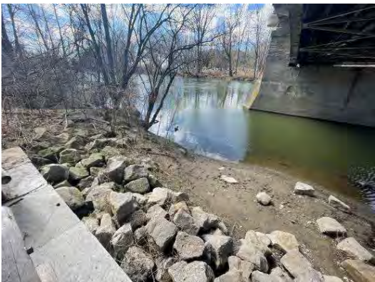
The east shoreline has been partially stabilized with rock protection in the vicinity of the pier and abutment (above). Culvert Outlet No. 5 is shown below and is immediately south of the bridge.
