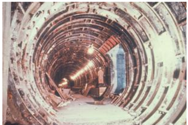
Figure 2. TTC Subway tunnel
