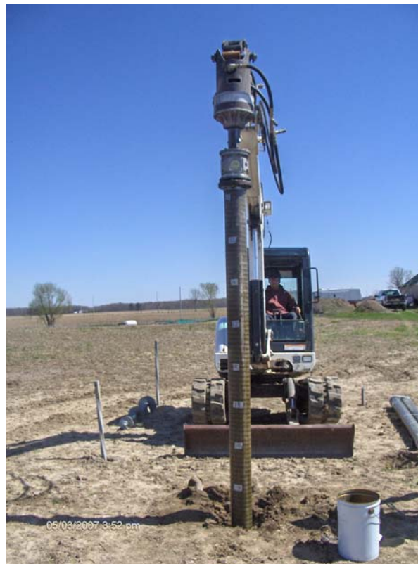
Fig. 5.b. FRP-G-HSP installation (internal SS175 shaft – external FRP 3m tube).
