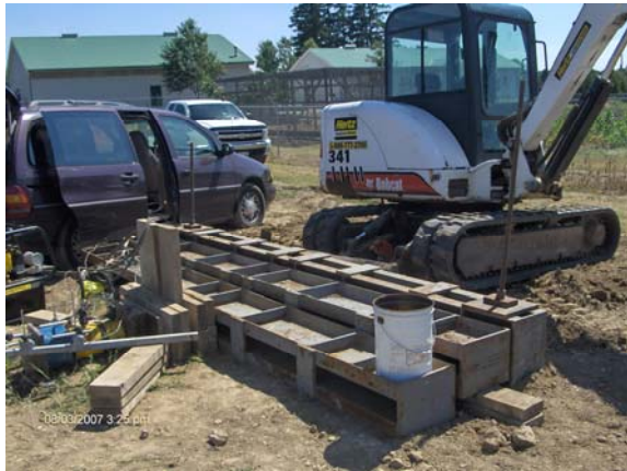
Fig.12.a. Lateral loading setup
