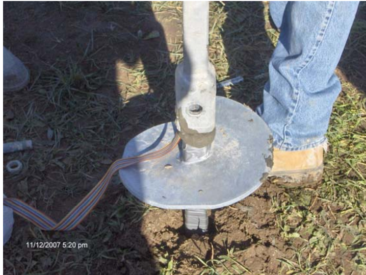
Fig.5.a. Typical preparation of lead section – extension connection
