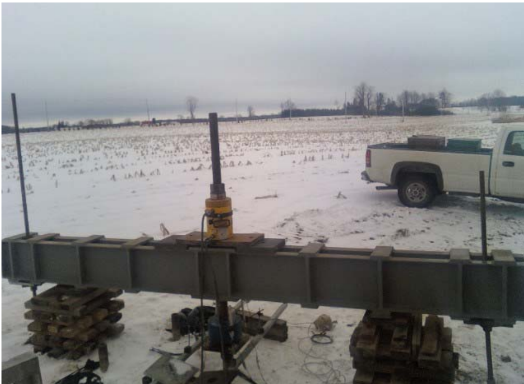
Figure 7. Tension Load test setup
