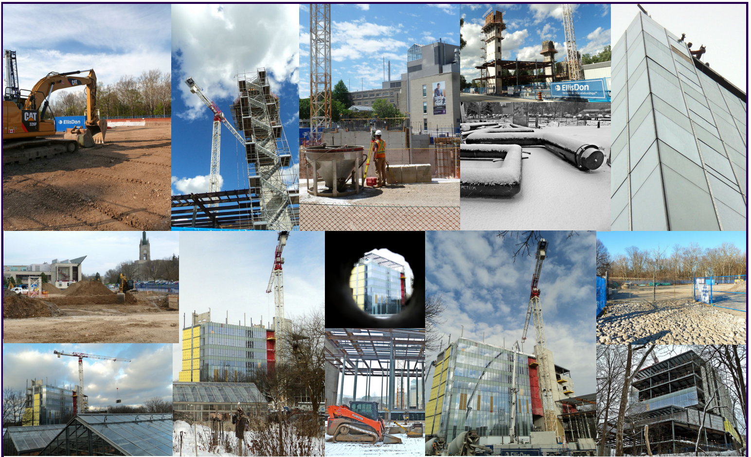
Construction of Western Interdisciplinary Research Building in 2016
