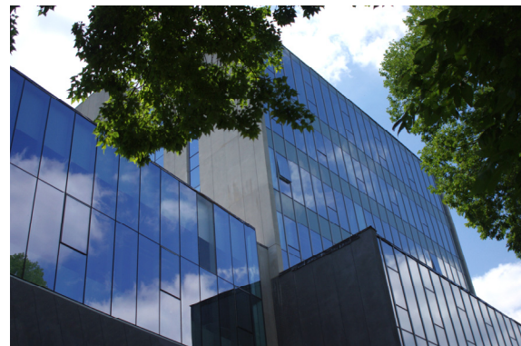
Western Interdisciplinary Research Building—river side
