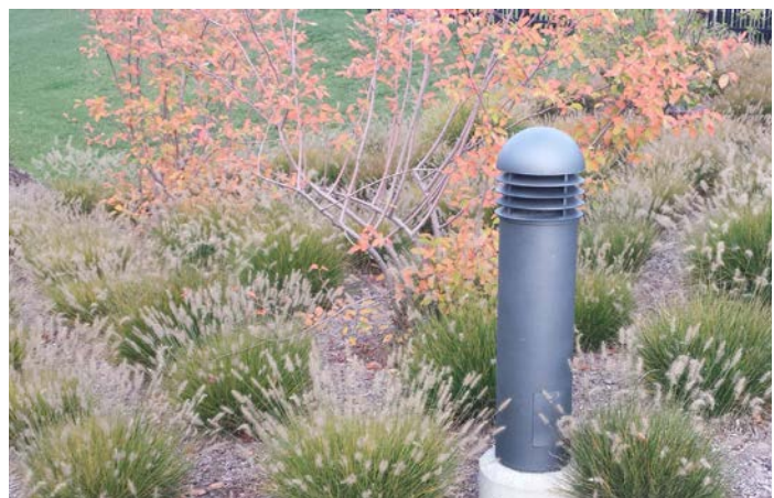
Figure 33. Bollard lighting at Ontario Hall Residence. (Source: Western University)
