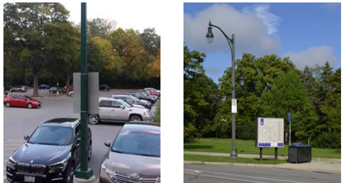
Figure 30. Existing light standards at Talbot Parking Lot (Left) and University Drive (Right). (Source: Western University)
