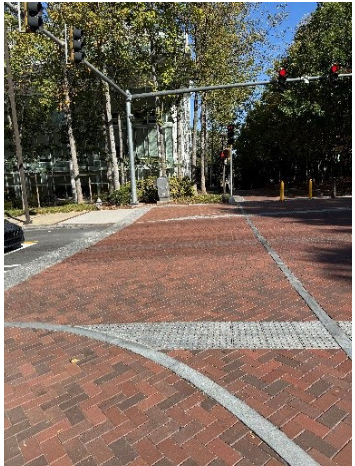
Figure 67. Tactile warning strips mark the raised intersection of a pedestrian and bicycle only street at Georgia Tech where it meets a standard street (Source: Nelson Nygaard)
