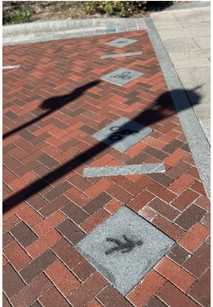
Figure 82. Custom granite pavers mark pedestrian and bicycle areas on Atlantic Drive at Georgia Tech, a core street converted to pedestrian and bicycle only use (Source: Nelson Nygaard)
