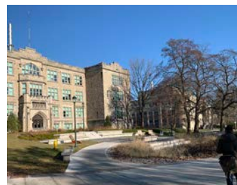
Figure 10. Kent Drive North (Source: Perkins&Will)
