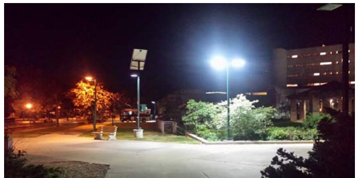
Figure 31. Difference between LED and High Pressure Sodium fixtures on Oxford Drive. (Source: Western University)
