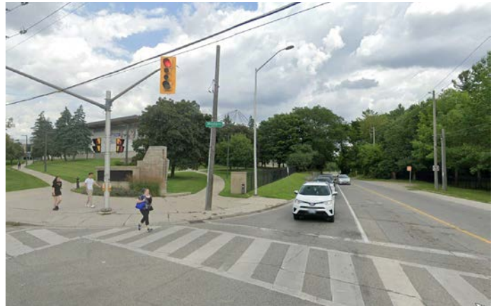
Figure 85. Philip Aziz Avenue at Western Road Gateway today
