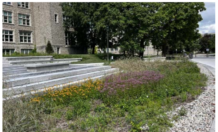
Figure 15. Rain garden in front of Physics and Astronomy building (Source: Western University)
