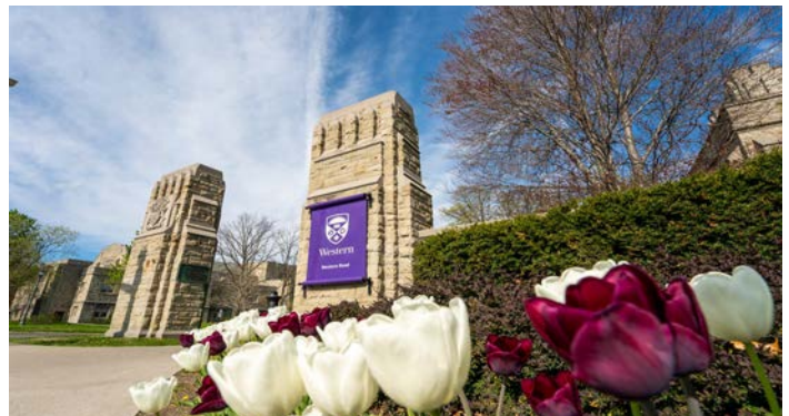
Figure 46. Campus gateways at Lambton Drive at Western Road
