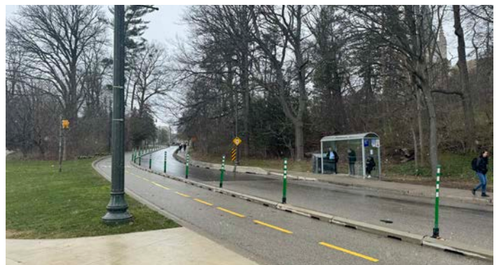
Figure 39. Two-way cycle track on Middlesex Drive near Perth Drive
