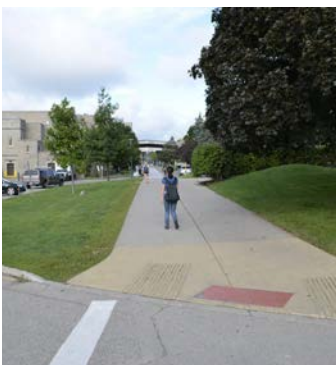
Figure 26. The bright red plates and yellow concrete ramps located at the edge of road crossings provides aid for the visually impaired. (Source: Western University)
