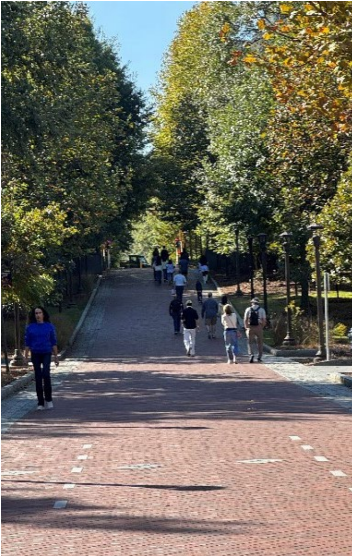
Figure 81. Custom granite pavers mark pedestrian and bicycle areas on Atlantic Drive at Georgia Tech, a core street converted to pedestrian and bicycle only use (Source: Nelson Nygaard)
