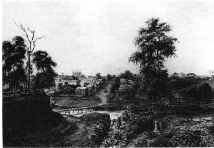
View of the Court House and the York Street foot bridge, circa 1850, by John Herbert Caddy.
