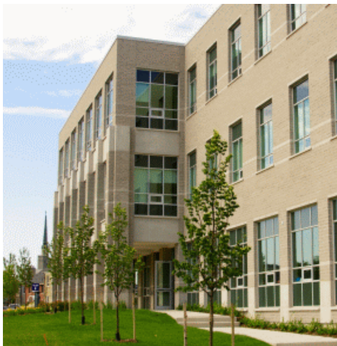
Support Services Building, Western Road
