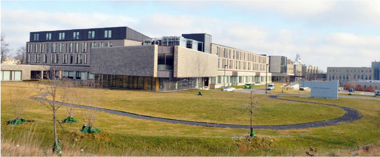
Western Road Development Site 1
